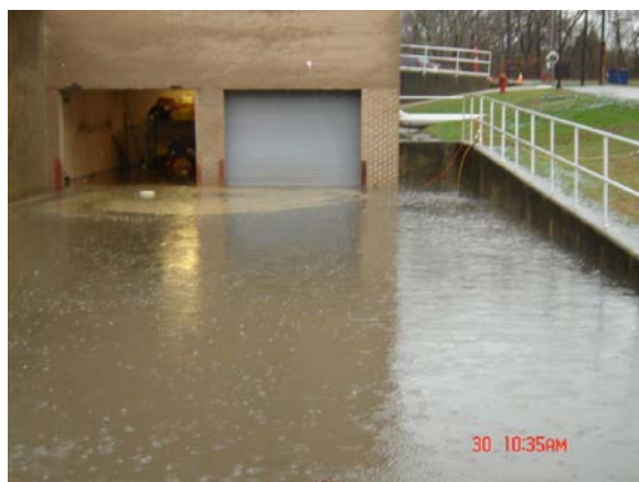
Figure 23: Westerly's lower garage filling with overflow from the overwhelmed plant uphill on March 30 th , 2010. Eight feet of water eventually found its way to this low spot. (Westerly)
