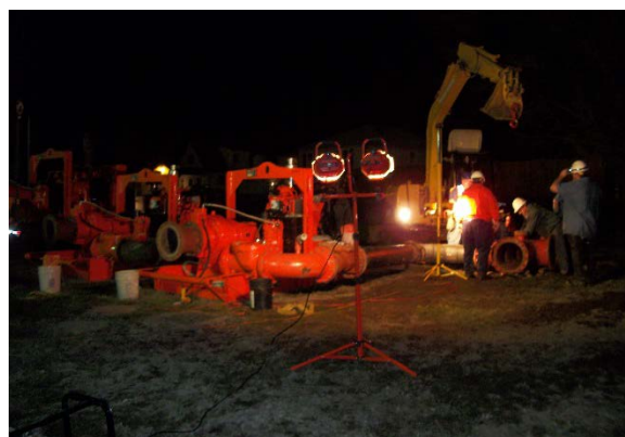
Figure 20: Bypass pumping being assembled at the Pontiac Avenue Pumping Station. (Veolia Water)
