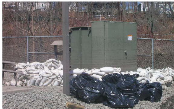
Figure 11: With flood waters long gone came remnants of frenzied attempts to sandbag critical components at the West Warwick Regional Wastewater Treatment Facility. (RIDEM)
